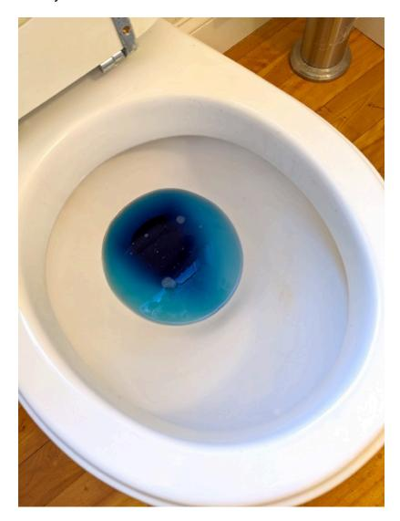
The water in p-traps can and does evaporate. If the water level drops below the top arch of the "u", then gas can start to drift up into your home.
